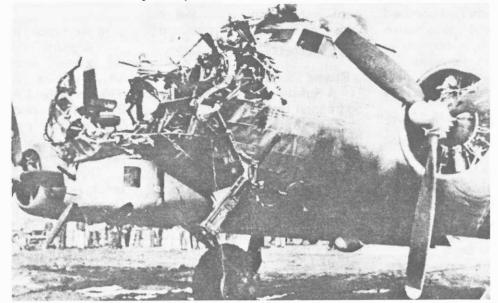
This B-17 may look unflyable, but it carried its crew from the skies over Cologne, Germany, to its home base in England. An anti-aircraft shell exploded in the Fort's nose at an altitude of 30,000 feet, knocking out navigational equipment, the plane's oxygen system and hydraulica.
