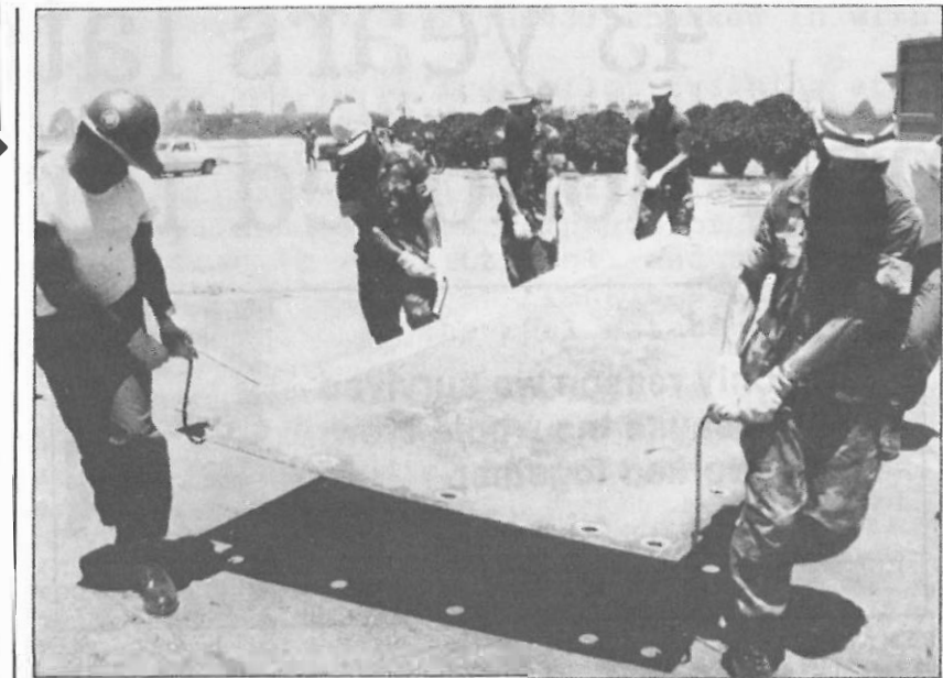
New resin-transfer molding techniques from the Naval Civil Engineering Laboratory make for better airport runway repair kits. In the picture, a fiberglass-reinforced plastic panel is moved into place to cover a bomb crater.
